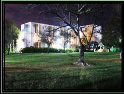
Antonio Ferré Building – Home of the Department of Geography and Regional Studies
